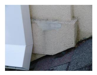
Remove debris and clean shingles and siding. Cut back EIFS a minimum of 8" above roof surface, patch EIFS, install metal roof-to-wall flashing with reglet or termination bar set in water-cut-off-mastic. Install backer-rod and compatible sealant.
