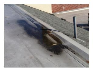
Install backer-rod and sealant to block transition vent extend ten feet beyond area of ponding water.
