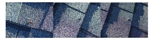
Remove protruding fasteners, apply compatible roofing cement.
