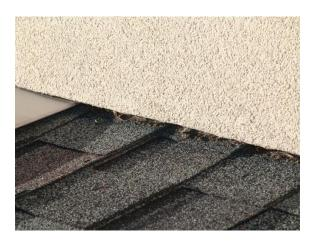
Remove debris and clean shingles/siding; install backer-rod and compatible sealant.
